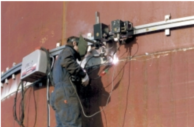
Aluminum Semi-Flex Rail (AFR) for large diameter applications down to a minimum radius of 15' (5 m). (Page 4)
